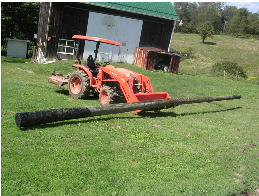
new HF antenna. I got the hole dug and the phone pole tarred on both ends. Using the tractor I placed the phone pole close to the hole it will be planted in. This is a lot bigger project than I had anticipated! I **will** get this new HF antenna together, it is just going to take a little more time than my original plan called for.
