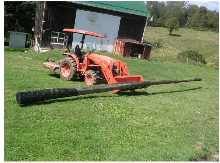
new HF antenna. I got the hole dug and the phone pole tarred on both ends. Using the tractor I placed the phone pole close to the hole it will be planted in. This is a lot bigger project than I had anticipated! I <u>will</u> get this new HF antenna together, it is just going to take a little more time than my original plan called for.
